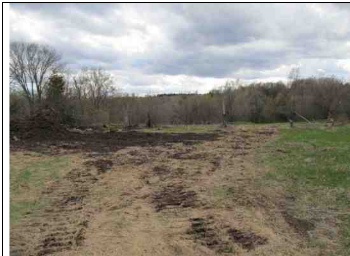
41. SGT pt 15. House removal location, toward south.
