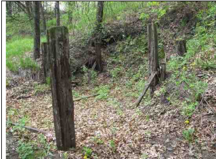
24. OW2 pt 33. Old building posts to be removed.
